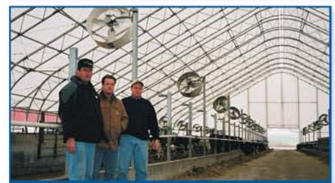
"The one benefit we didn't plan on is that these structures would protect our animals from a tornado!" - Allen Abel
