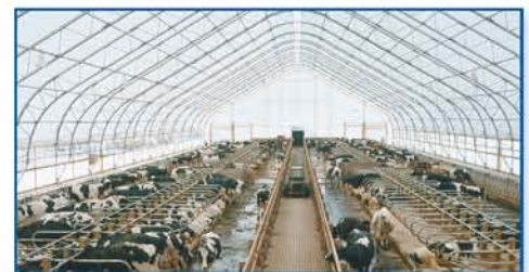
An additional 20 feet was added onto one of the free stall barns to increase the length to 380 feet. Install of the two buildings was completed in just 17 days
