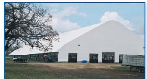
Two new Cover-All TITAN buildings were manufactured and delivered to the site in eight days.
