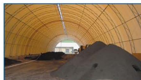
Condensation is exhausted through the 10 inch center ridge vent
