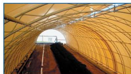
The building covers two 270 foot windrow piles that are each 12 feet wide by 5 feet high
