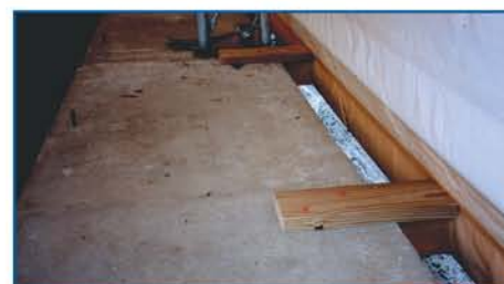
The 3 inch low-level air intake helps to create natural air circulation
