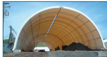
Cover-All Arch building series to cover 55 foot by 290 foot composting platform
