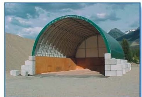
A 42' x 60' Arch stores salt at Blue River, BC
