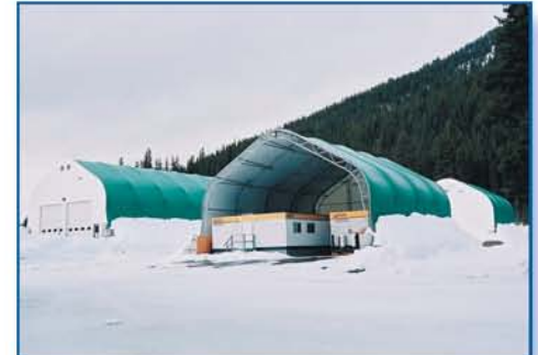
Three TITAN's house equipment and salt at Allison Pass, BC
