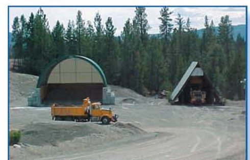
According to operators, the Cover-All buildings are easier to dump salt in than conventional structures
