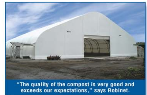
A large overhead door allows for the passage of a shovel.
