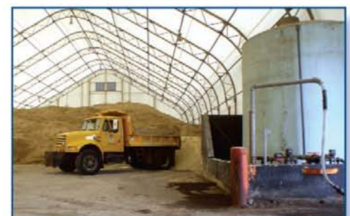
The building is designed with two doors on either side to allow for efficient loading of materials and stops at the liquid tanks.
