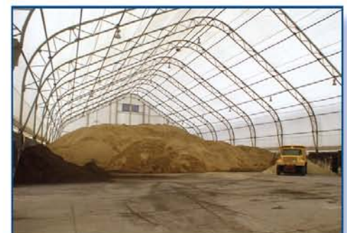
The Cover-All building houses 10,000 tonnes of winter sand and 1,000 tonnes of pure salt.
