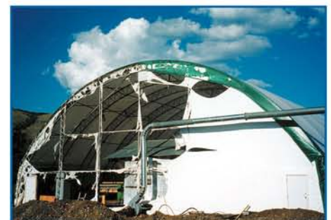
When Cover-All's unique DuraWeave® cover is exposed to fire, it simply burns away and extinguishes itself.
