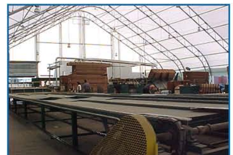
The 120' wide x 140' long Cover-All® TITAN® houses the new plant.
