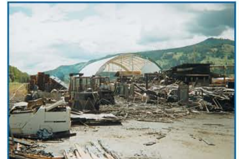
The fire destroyed the wood warehouse 15 feet away from the Cover-All® building.
