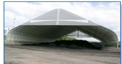
Once the foundation was complete, construction moved very quickly.
