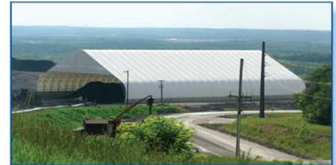
The 160' wide by 260' long (48.7m x 79.2m) Cover-All® TITAN® building is used for the storage and drying of coal.
