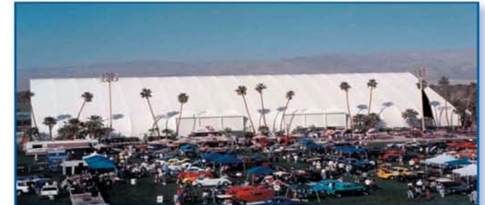
The 160' x 300' TITAN building is nearly 60' high and offers 48,000 ft 2 of clear-span space
