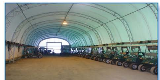
Falcon Lake Golf Course houses 60 carts inside their Cover-All® building which has resulted in a lot less maintenance.
