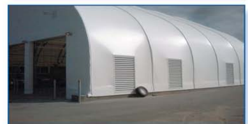
Extensive ventilation was installed to exhaust engine fumes
