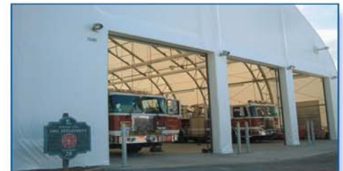
The 14' x 20' electric bay doors provide an ample passage way for emergency exits
