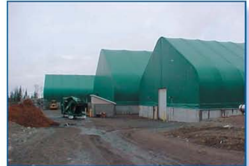
The four TITAN buildings were placed on a 4' thick x 5' high concrete foundation.
