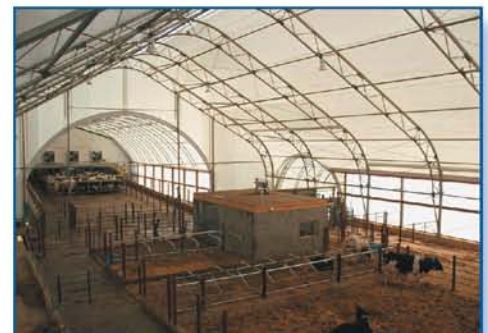
The 90' x 120' barn for close-up cows is connected to the 50' x 80' holding area.
