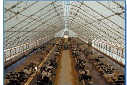
Hood Dairy Farms 100' x 460' free stall barn attached to a 30' x 96' crosswalk.
