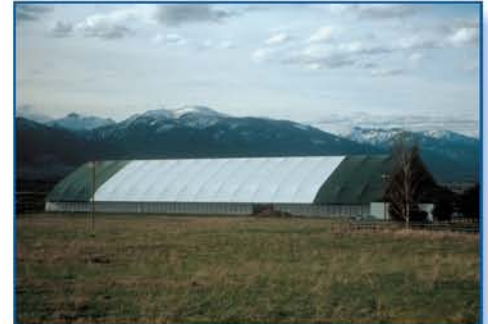
Installation of the 43,200 sq. ft. free-stall dairy required only 10 days
