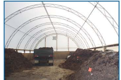
The Cover-All® polyolefin fabric cover is not affected by the corrosive environment.
