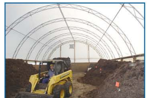
The clear-span design of a Cover-All® building allows ample room to operate machinery and establish compost windrows.
