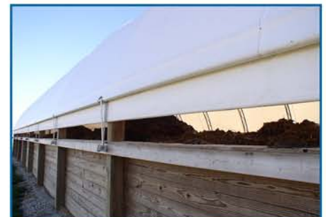
2' side curtain walls provide natural ventilation and eliminate condensation inside the building.
