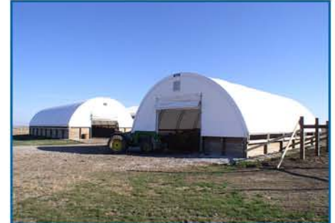
Hy-Line's composting process takes place in two 40' wide x 60' long Cover-All® buildings and one 40' wide x 80' long Cover-All® building.
