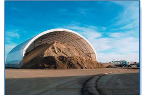
Cover-All Arch buildings are used for salt and sand storage at 29 locations across central Alberta
