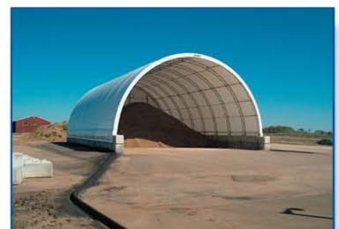
A curb runs along the asphalt pad keeping water from seeping into the ground
