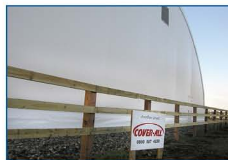
"From breaking ground to riding inside, the entire building installation took only five weeks!" says Brian.
