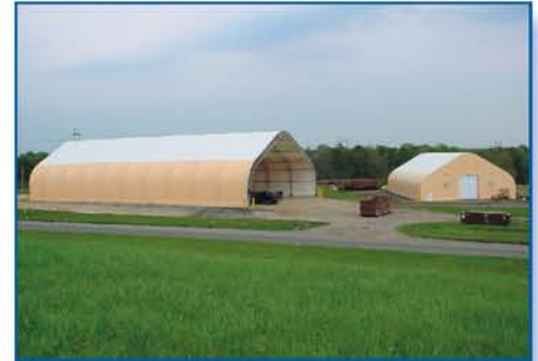
Two Cover-All TITAN buildings warehouse equipment and salt and sand at the landfill in Tinton Falls, NJ
