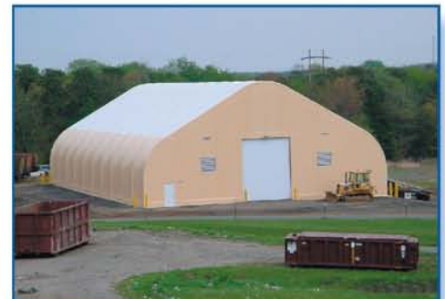
The 80' x 150' TITAN stores equipment used to maintain the 900-acre landfill.
