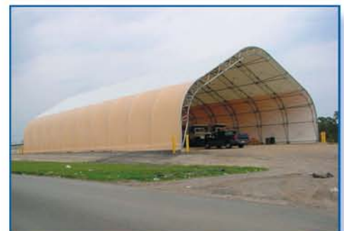
The 70' x 150' TITAN is ideal for salt and storage. The open end allows easy access for loaders and sanders.
