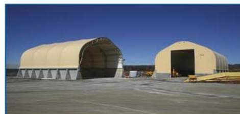
"The average time for a crew of four to install a 60' (18.2m) wide x 90' (27.4m) long building is just seven working days," says Ben Hogervorst, president, CABS NY.
