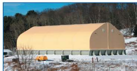
The Cover-All® TITAN® buildings used to store salt range in size from 50' (15.2m) to 60' (18.2m) wide and 90' (27.4m) long.
