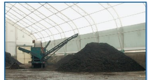
The new 90' x 220' TITAN™ building addition is utilized to screen and remove further residual, as well as added storage
