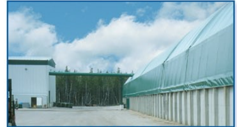
The 72' x 440' Arch™ and 90' x 220' TITAN™ building were positioned on 10' high concrete containment walls
