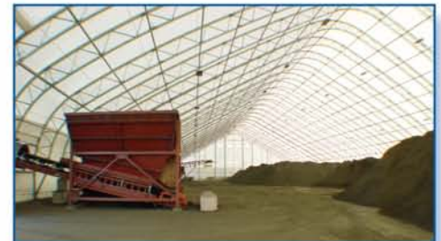
"The ability to allow light into the facility has minimized the need to turn on the lights during the day which has been a nice change from an energy savings perspective," says Krout.
