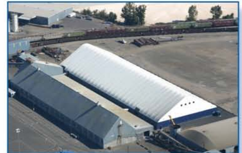
The 72,000 ft 2 (6,689m 2 ) storage facility was installed in six weeks.
