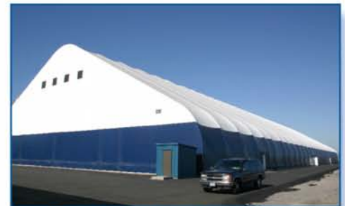
Eight 4' by 4' (1.2m x 1.2m) mesh vents were installed in the end walls to provide the required air circulation.
