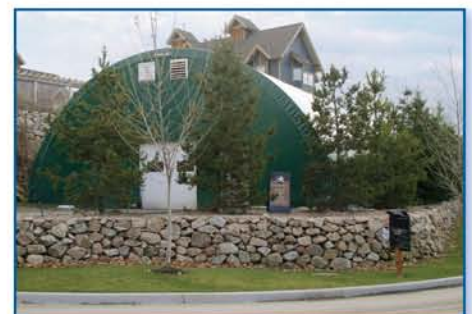
The green color of the building blends in well with the surrounding environment.
