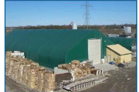
Rancor Wood Recycling houses its operations in four Cover-All® buildings.
