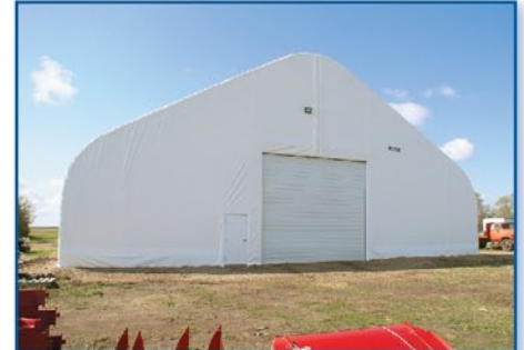
Redekop chose a 70' wide x 80' long Cover-All® TITAN® for equipment storage.
