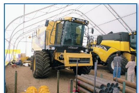
The fire retardant DuraWeave® membrane cover allows natural light to penetrate the building.
