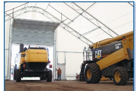
The 18' x 16' overhead door allows quick and easy access to equipment.
