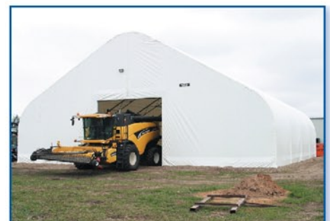
The Cover-All building provides protection for machinery and workers from the elements during R & D tests.
