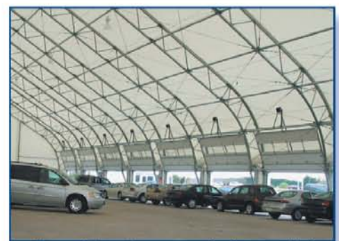
The ten 14 foot doors across the front provided the dealership with the flexibility they needed.
