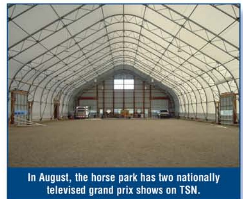
"They're the most cost effective building out there right now and that's why we keep adding more, because there are no drawbacks to the cost effectiveness," says Chris Pack.
