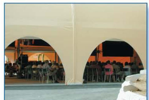
Scalloped openings that run along the side of the building are ideal for entranceways and ventilation
