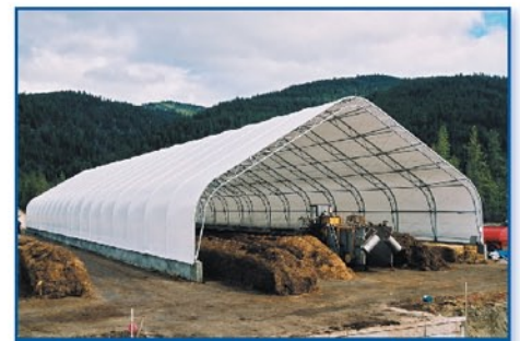
Open ends and a center ridge running along the ceiling aid in the exhaust of compost steam.
