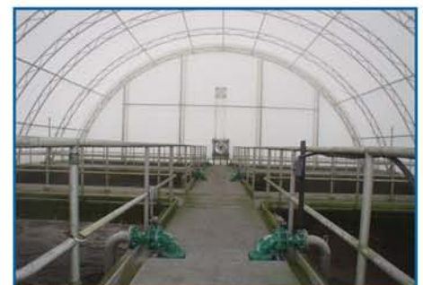
Natural light penetrates the membrane cover, eliminating the need for artificial lighting.
