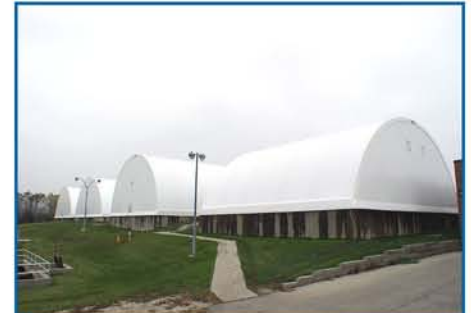
The four 62' wide x 62' long Cover-All buildings cover two sludge tanks each.
