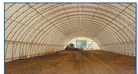
The Cover-All Arch will be disassembled and relocated to other sites once the job is complete.
