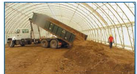
Hot pockets of contaminated soil are identified and transported to the Arch for composting.
